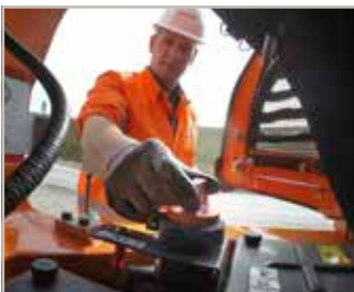
Battery cut-off switch
