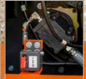
Primary filter head with ETP-Switch
